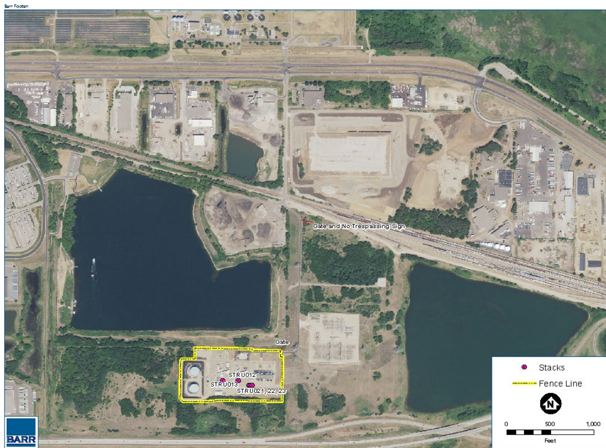
Figure 2 Xcel Energy Blue Lake Plant North Entrance Gate and Posted Signage
